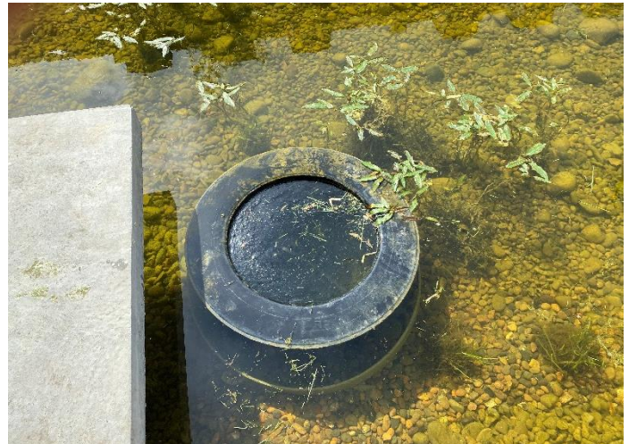
Figure 2: installed in the filter bed Skimmer 360°
